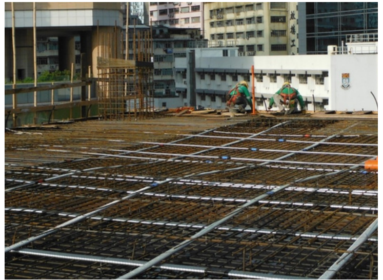
ABOVE: A typical PT Concrete slab of Trade and Industry Tower - Hong Kong (Office & Headquarters)
